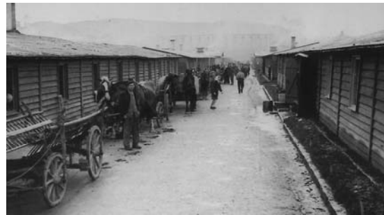
Today's „Gartenstraße“ („garden street“) in Gusen, shortly after Gusen I und II had been freed by US troops, in May 1945 © National Archives and Records Administration (NARA), Washington, D.C.
